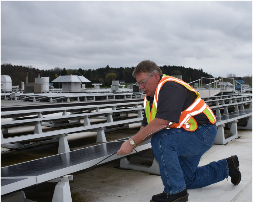
Jamestown Engine Plant electrician Fred Gable inspects the solar panel connections at Cummins’ roof-top solar array at Jamestown, New York (U.S.A.). The plant is one of the locations where the company has added renewable sources to its energy mix.
