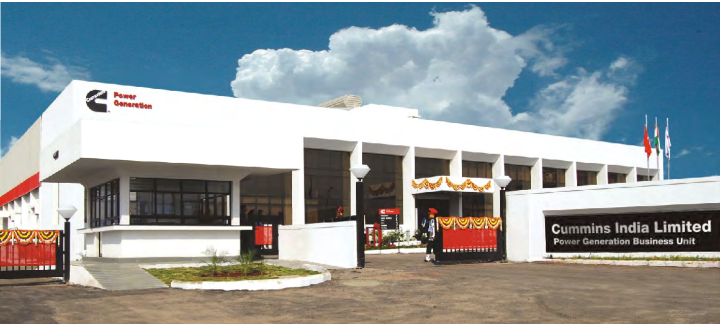
New state-of-the-art manufacturing facility of the Power Generation Business Unit at Pirangut. Set up to manufacture small generator sets.
