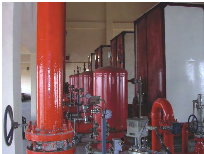
Firepump Installation powered by Cummins V28 engines
