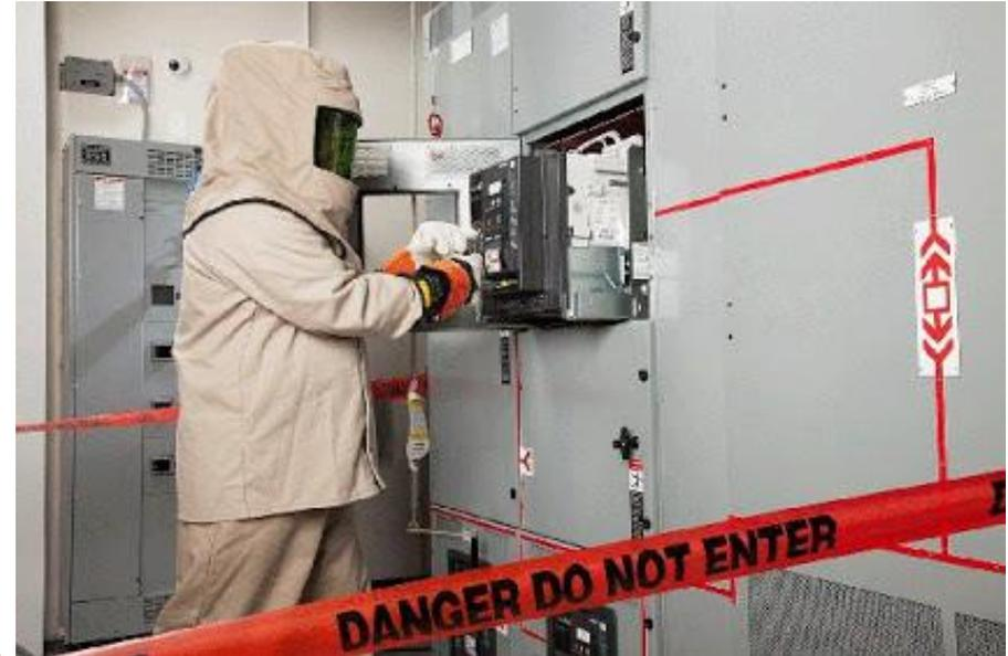
Allows a worker to set a circuit breaker electronic trip unit or protective relay to operate faster should an arc fault occur while the worker is working within the protected zone
