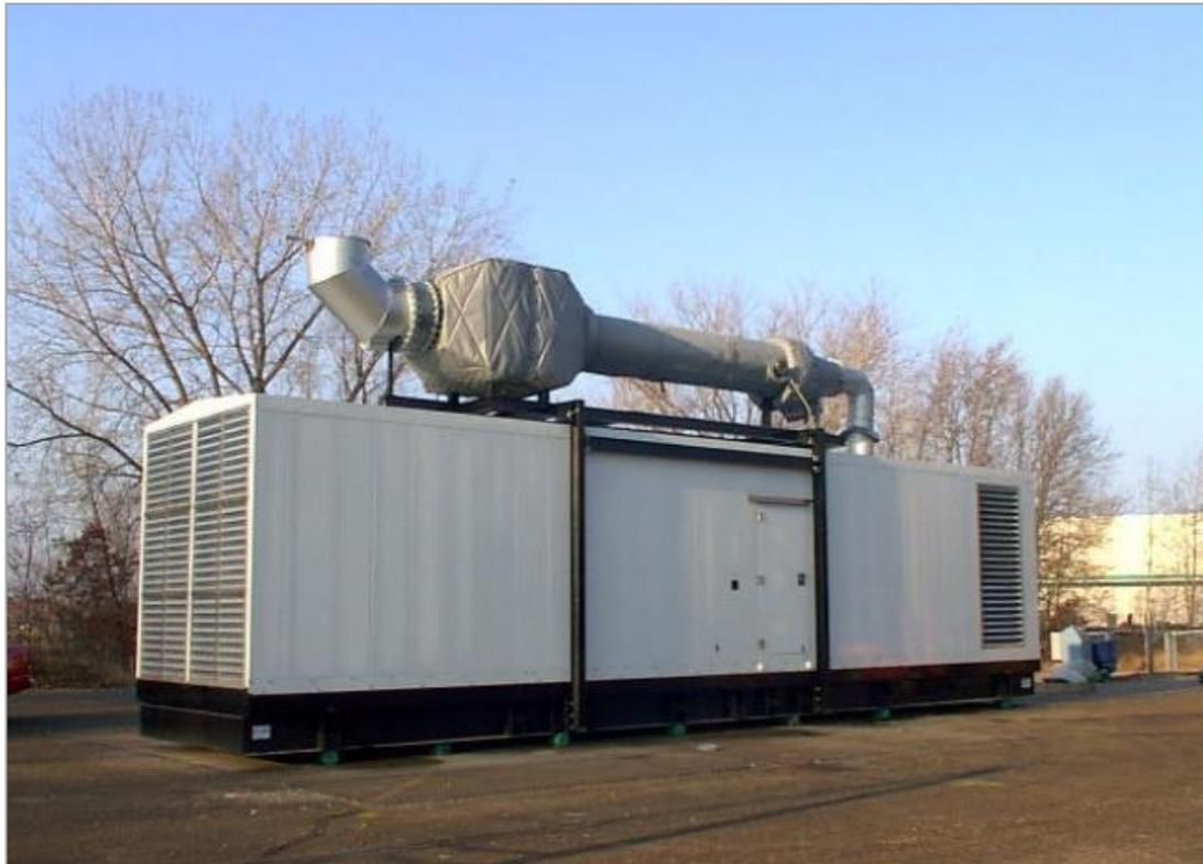
Diesel Particulate Filter (DPF) can reduce Particulate Matter
