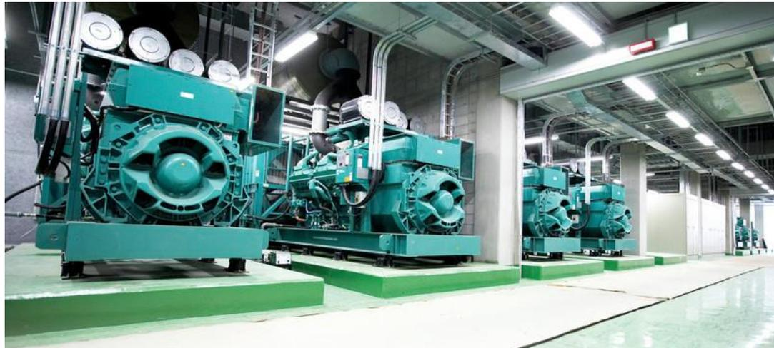
Standby power system including seven C2000 D6 (2000 kWe) generator sets.
