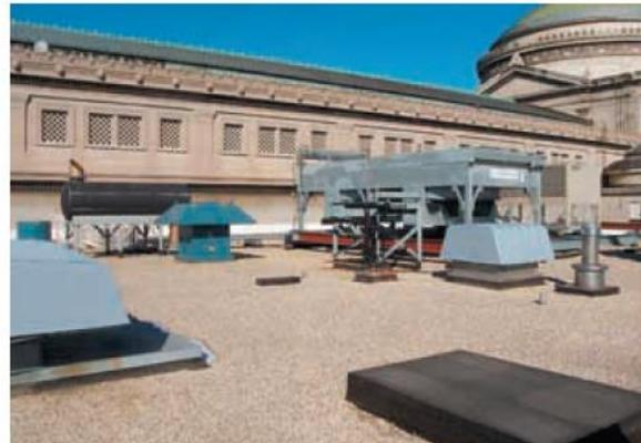
The lean-burn engine's radiator and critical exhaust silencer are roof mounted.
