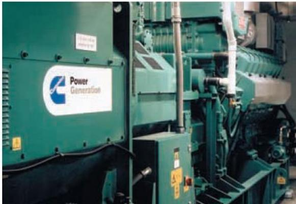
The Cummins Power Generation lean-burn generator set produces up to 1.75 MW of electricity and 4,000 pounds of steam per hour in a CHP application.
