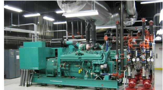
**Application:** Emergency standby system including two DQGAA (1250 kWe) and one DQGAB (1500 kWe) provided by Cummins.
