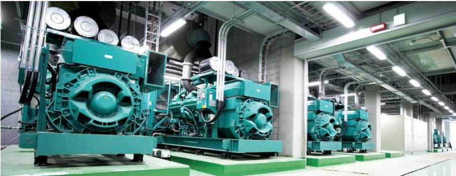
**Application:** Standby power system including seven C2000 D6 (2000 kWe) generator sets provided by Cummins.
