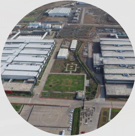
Cummins Megasite Manufacturing Campus
